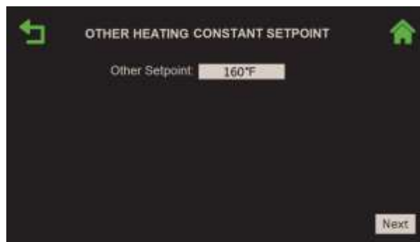
Figure 2-56: BST Manager – Other : Other Heating Constant Setpoint Screen
