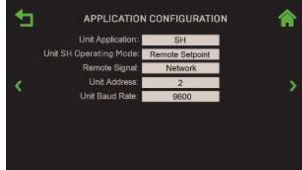
Unit SH Operating Mode = Remote Setpoint
