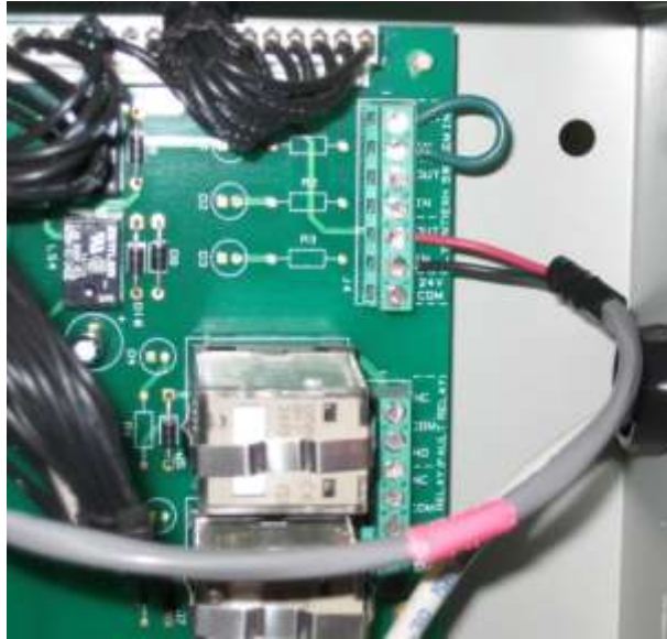
Figure 2-14: Sequencing Isolation Valve Installed
