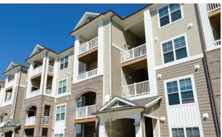
Multifamily/ Apartment Buildings
