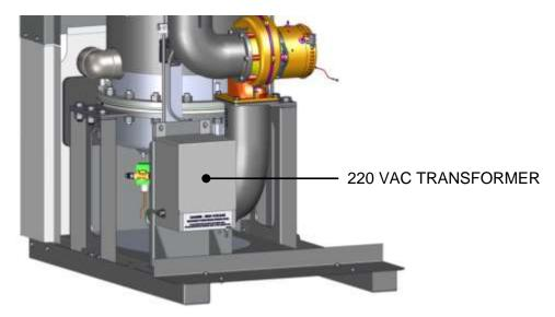
Figure 2.11-3: 220 VAC Transformer – Front and Side Panels Removed
