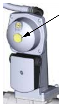
Figure 4-8. SSOV Gas Pressure Adjustment Screw Location
