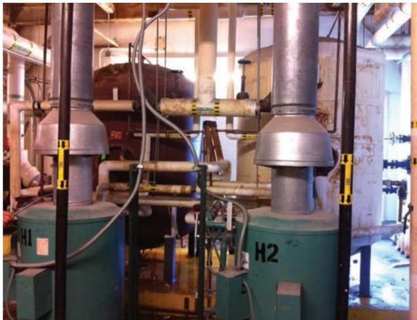
PHOTOS A and B. A mechanical room before (left) and after (right) tanked systems were replaced with tankless systems.
