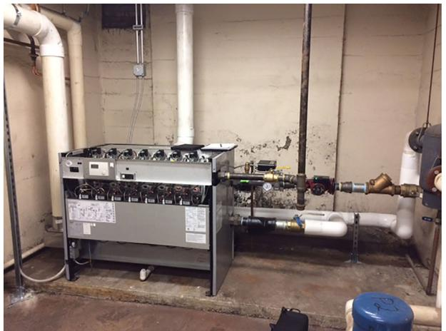
PHOTOS A and B. The first facility’s mechanical room before (left) and after (right) the installation of a Modulex EXT 1060 boiler.
