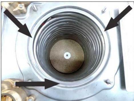
**Figure M: Clean Gasket Surface**
