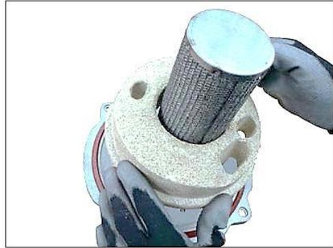
**Figure J: Install Thermal Insulation**
